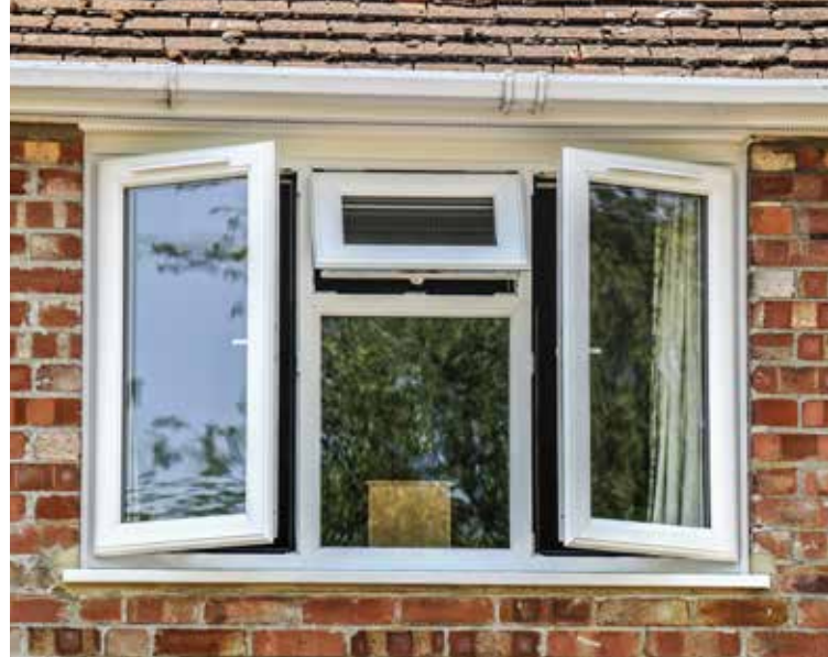
Trickle Vents installed through the window sashes
